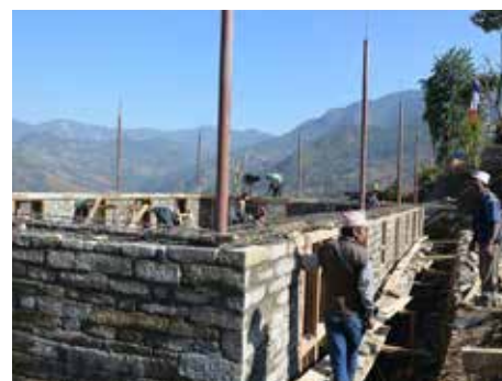
Walls almost complete!
