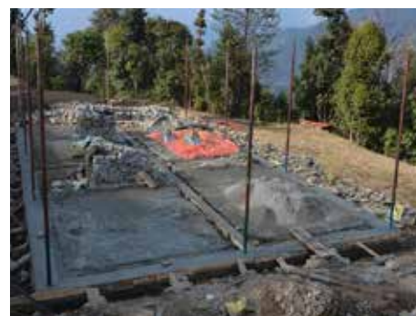
The foundation of Home of Hope
