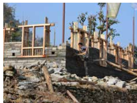
Window and door frames in place
