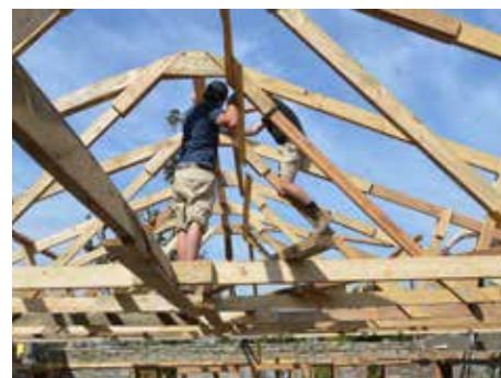
Roof frames made by Johan Magnusson
